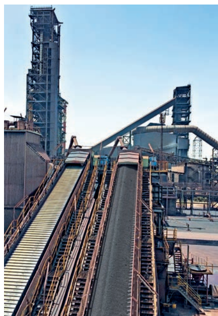
Conveying and cooling of pellets with AUMUND Pan Conveyor type KZB-K
