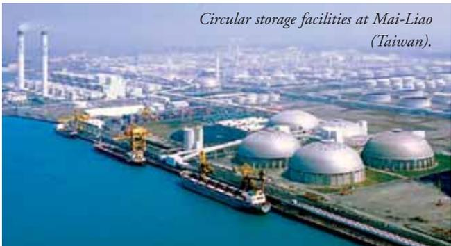
Between 1997 and 2003 a total of eleven domes were constructed nine of which are for coal storage with two dedicated to salt storage for the plastics process, at 120 metres diameter these were the largest circular storages in existence.
